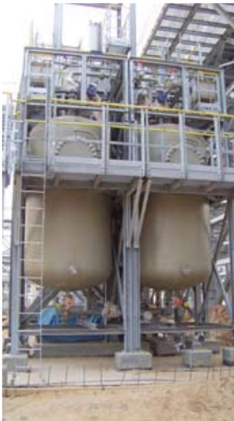
Figure 3: Two activated carbon modules are a major component of the modular candle filter plant in Turkmenistan.
