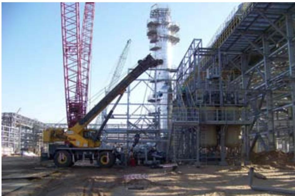
Figure 2: The modular construction principle enabled the BHS candle filter plant to be erected on site in a short space of time.
