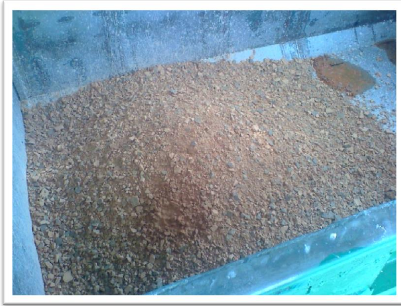
Figure 6: BHS Candle Filters, 2 x 100 m 2 , cake discharge
